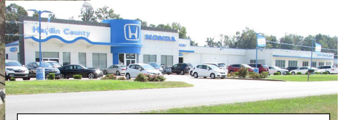
24,000 sq. ft. Commercial Building
