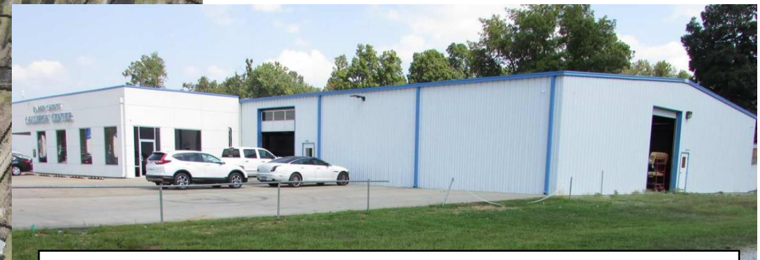
20,000 sq. ft. Commercial Building
